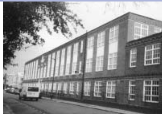
Figure 2 1926 addition to the school, fronting Grove Lane
